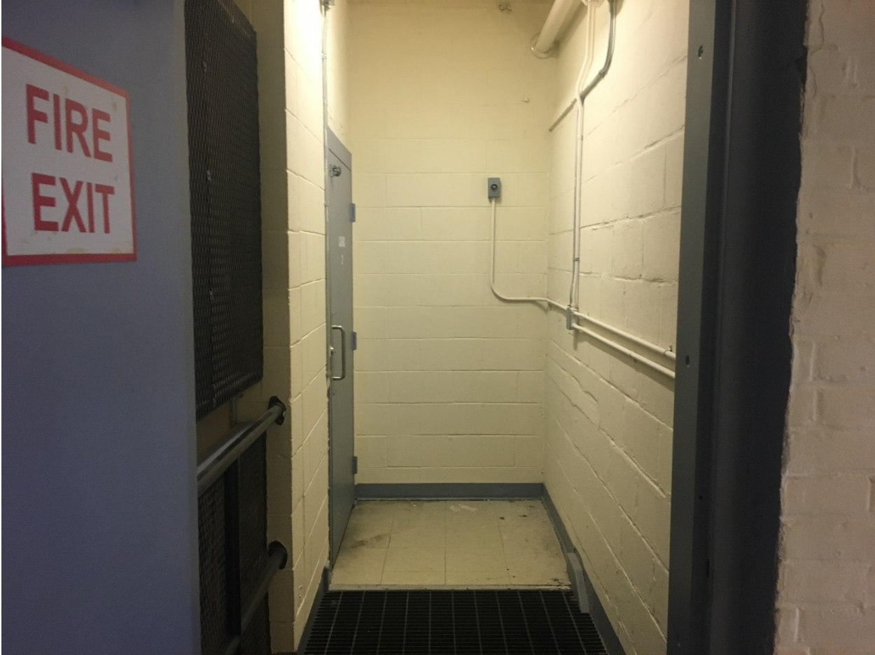
Photo 3: Bad site lines into units; door at the end of the hall, no window on door.
